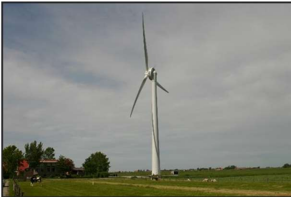
Figure 15 EWT 500 kW turbine
